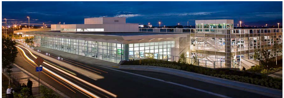
TSAIA CONRAC Facility
