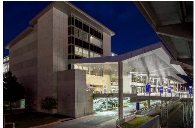
ABIA CONRAC Facility - Exterior
