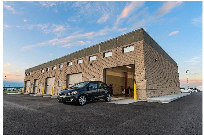
BIS Consolidated Quick Turn-Around Facility
